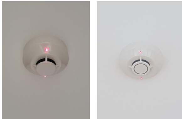
Smoke detector and thermal detector with alarm LED activated.
